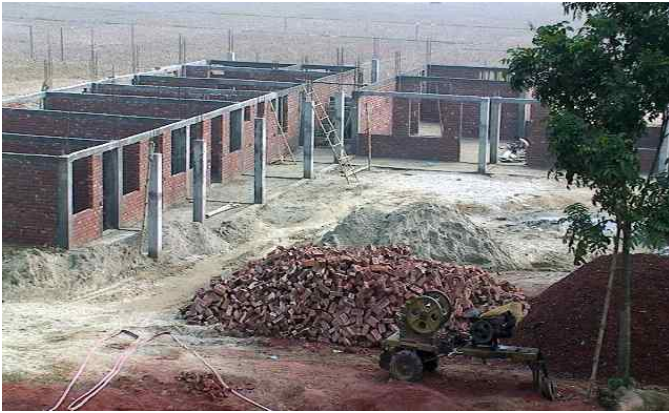
Our orphanage walls are taking shape
